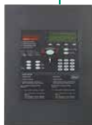
Fire Alarm Control panel
